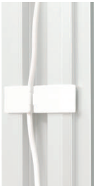
CLEAN CABLE MANAGEMENT
